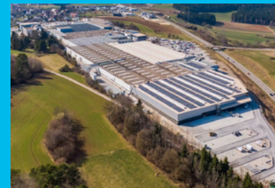
Photovoltaic system in Schopfloch
