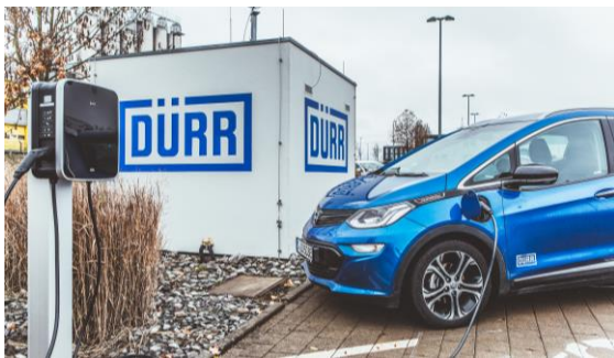
11| Charging station in Bietigheim-Bissingen (Germany) (Source: Dürr AG)
